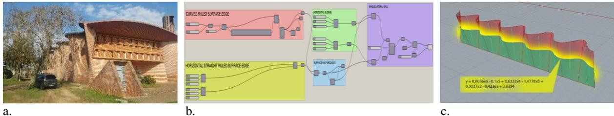
a. Figure 1: (a) The Church of Cristo Obrero, design and built by Eladio Dieste between 1956 and 1958 in Atlántida, Uruguay. (b) Algorithm developed in Grasshopper 3D in association with Rhinoceros 3D from 6<sup>th</sup> degree polynomials (c) extracted from the construction drawings.
